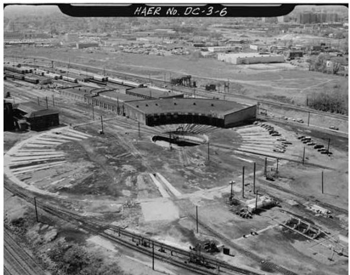
Aerial Photograph, Ivy City Roundhouse, 1977
