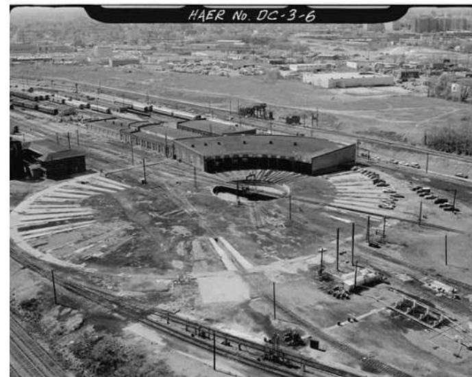
Aerial Photograph, Ivy City Roundhouse, 1977
