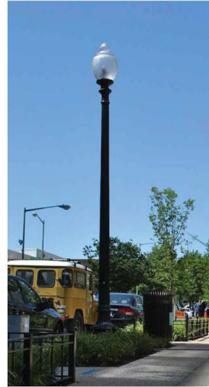
STREETLIGHT - (DDOT standard)
