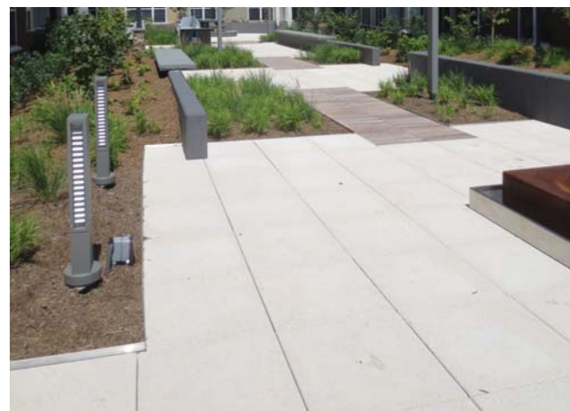
PRECAST CONCRETE PAVERS ON PEDESTALS
