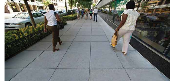
CONCRETE SIDEWALK - 3X3 SCORING PATTERN
