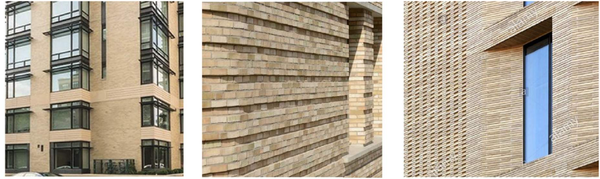
A BRICK MASONRY
