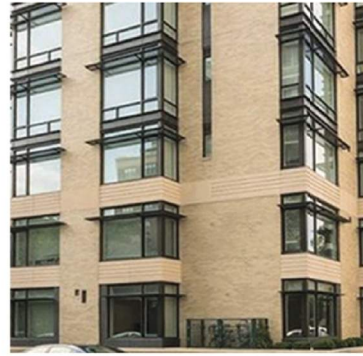
A BRICK MASONRY
