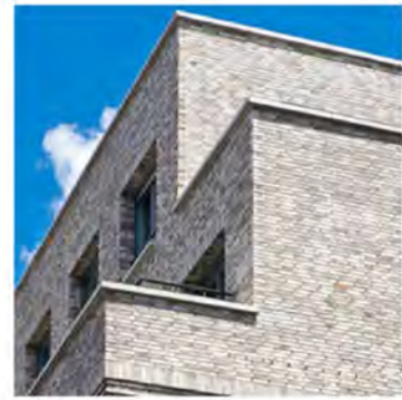
A BRICK MASONRY
