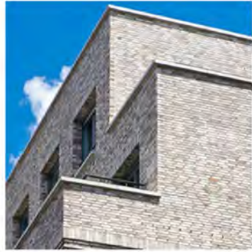
A BRICK MASONRY
