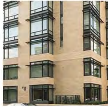
A BRICK MASONRY
