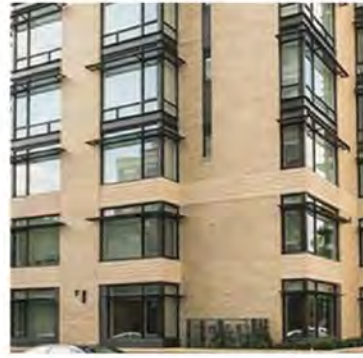
A BRICK MASONRY
