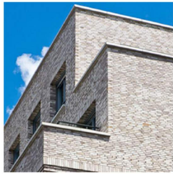
A BRICK MASONRY
