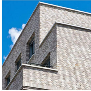
A BRICK MASONRY
