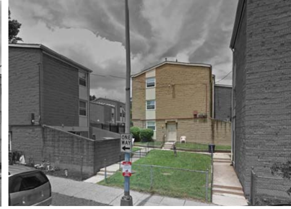
INTERIOR BUILDING NETWORK
