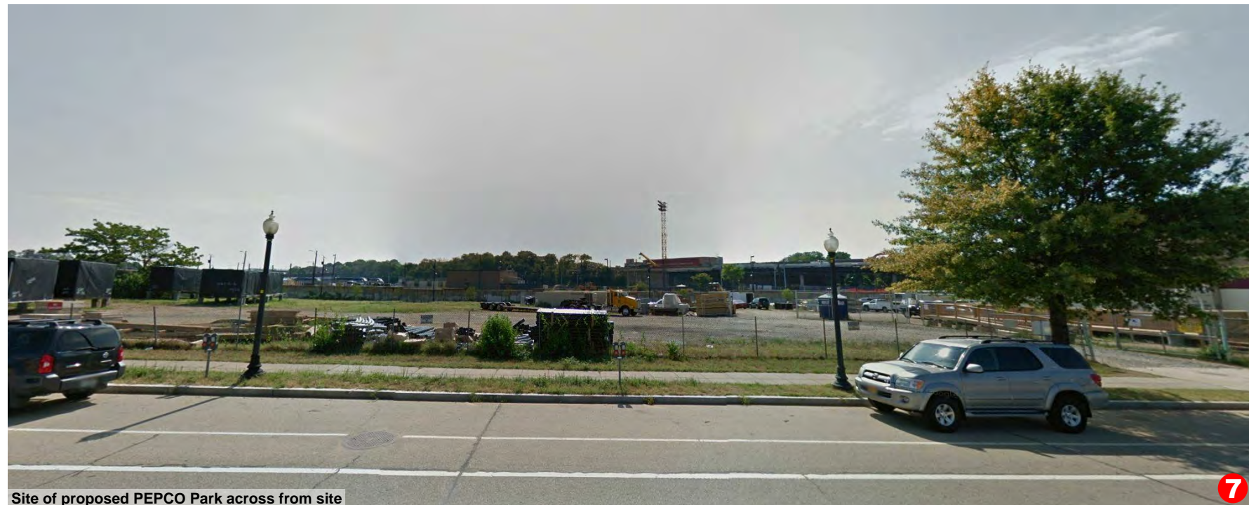
Site of proposed PEPCO Park across from site
