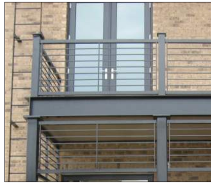
① STEEL BALCONY / RAILING
