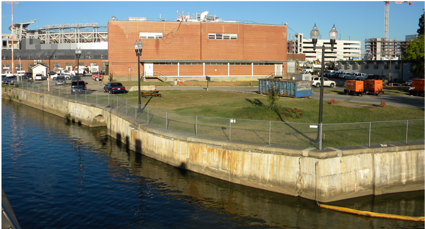
VIEW FROM ANACOSTIA RIVERWALK TRAIL - FACING NORTHWEST
