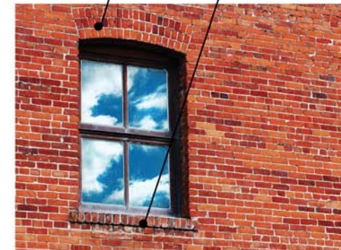
bowspring arch head or jack arch head, re: elv rowlock sill
