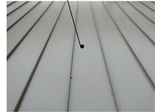
standing seam metal roof
