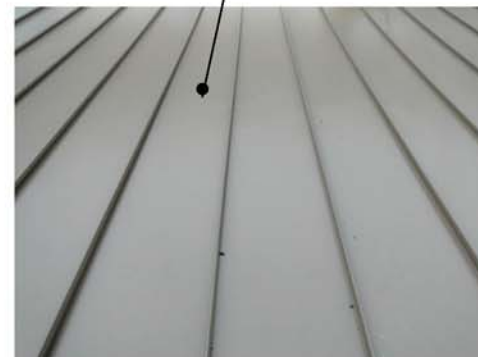
grey standing seam roof
