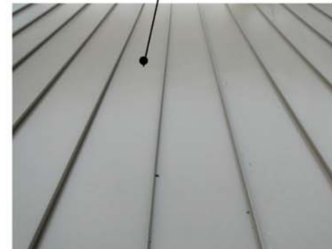
grey standing seam roof
