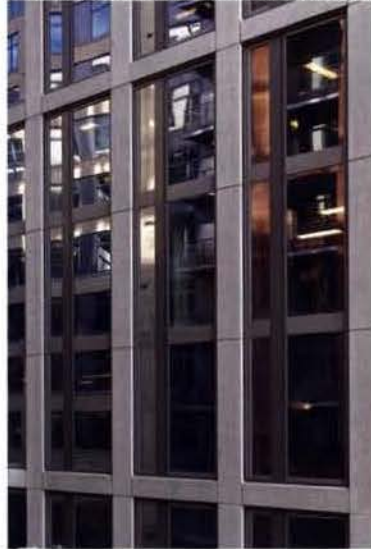
PRECAST CONCRETE WALL WITH WINDOW WALL
