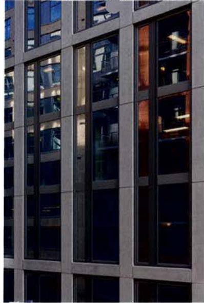
PRECAST CONCRETE WALL WITH WINDOW WALL
