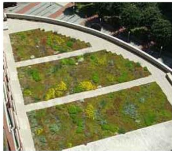
EXTENSIVE GREEN ROOF
