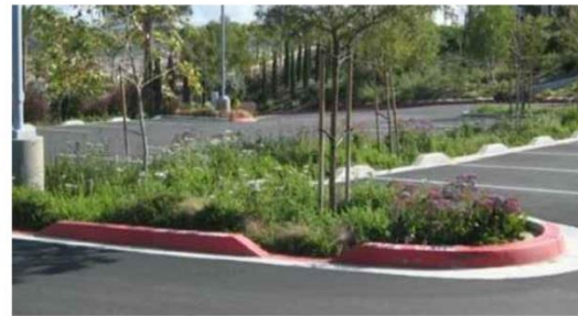
PARKING LOT BIORETENTION
