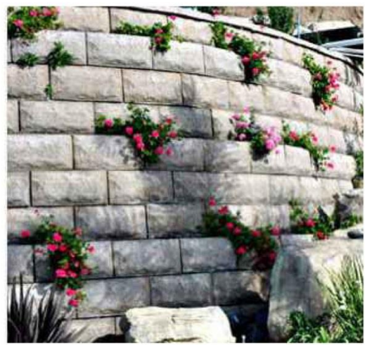
RETAINING WALL WITH VEGETATION INSERTS
