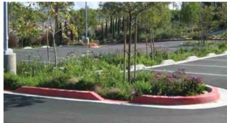
PARKING LOT BIORETENTION
