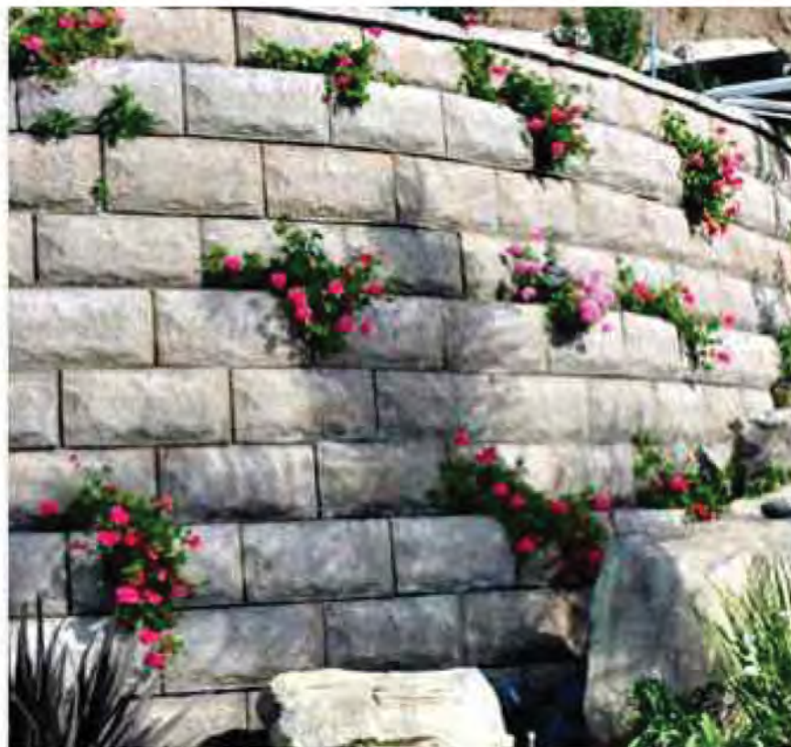
RETAINING WALL WITH VEGETATION INSERTS
