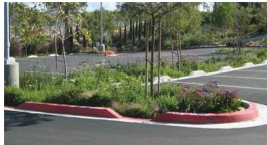
PARKING LOT BIORETENTION
