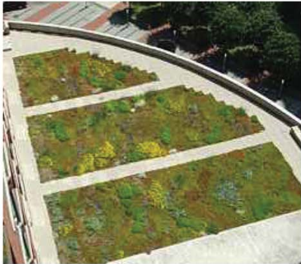
EXTENSIVE GREEN ROOF
