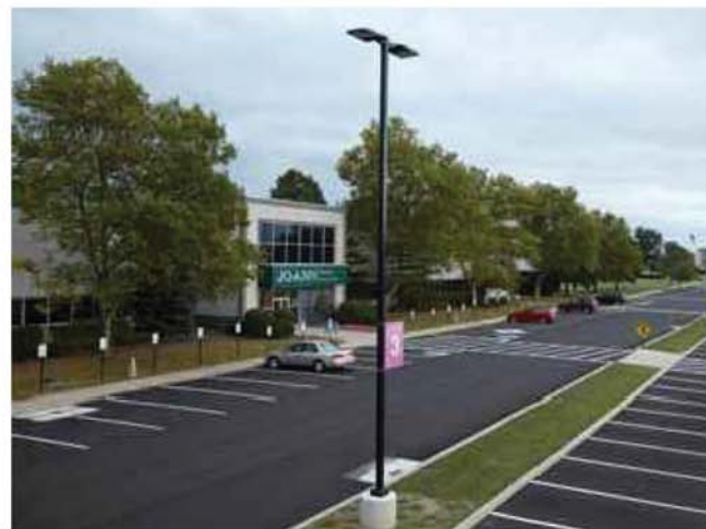
PARKING LOT LIGHTING
