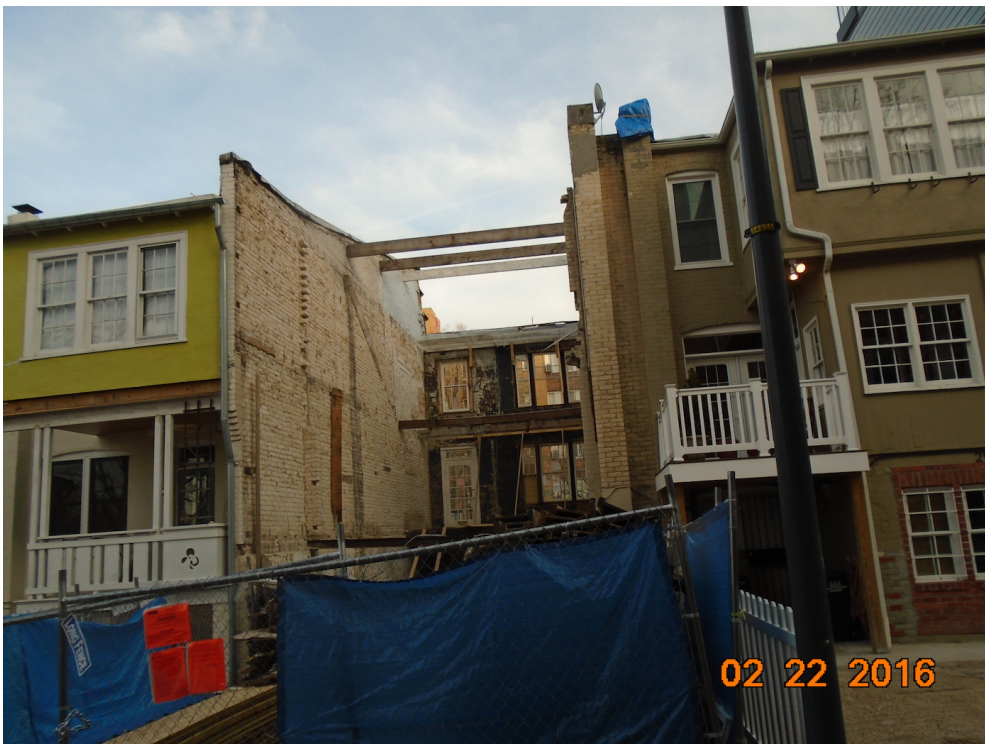
NEW HOUSING FOR NEW NEIGHBORS: One of two 18th Street row houses currently awaiting redevelopment.
