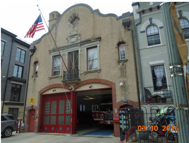
Firehouse next to 1761 Lanier Place
