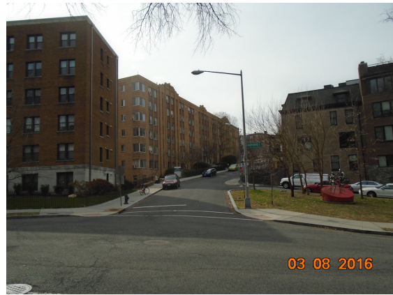
Park Crescent Apartments on 18th St.
