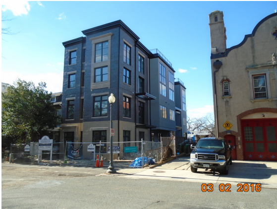
1767 Lanier Place: Lanier Station
