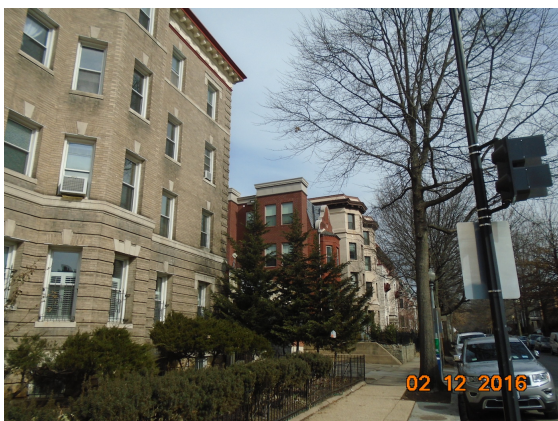
Lanier Place from Adams Mill Road
