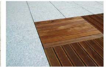
Pavers and Decking
