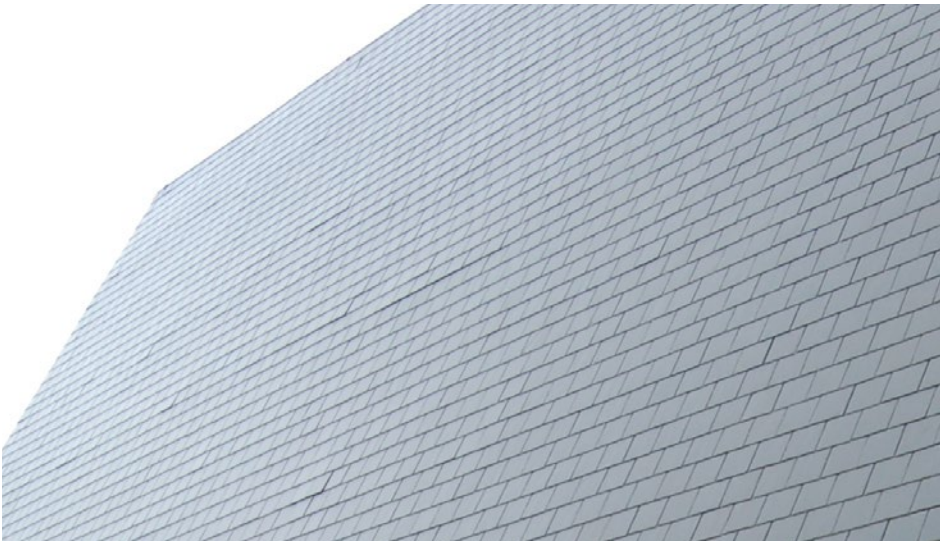
CHURCH - SLATE WALL CLADDING
