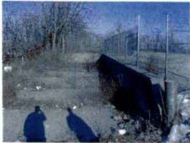
CONCRETE RETAINING WALL AND CHAINLINK FENCE
