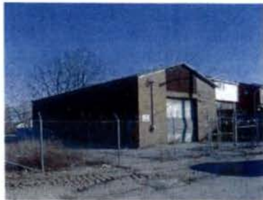
CHAINLINK FENCE AND EXISTING BRICK STRUCTURE
