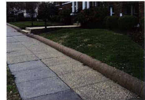
3) Restored concrete rolled curb
