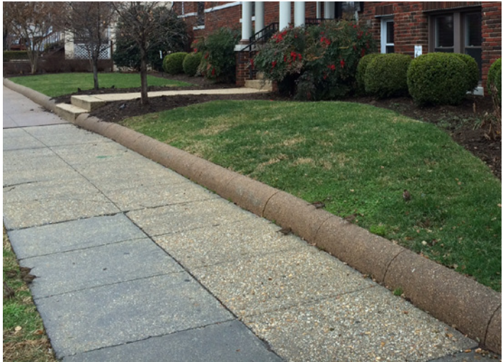
3) Restored concrete rolled curb
