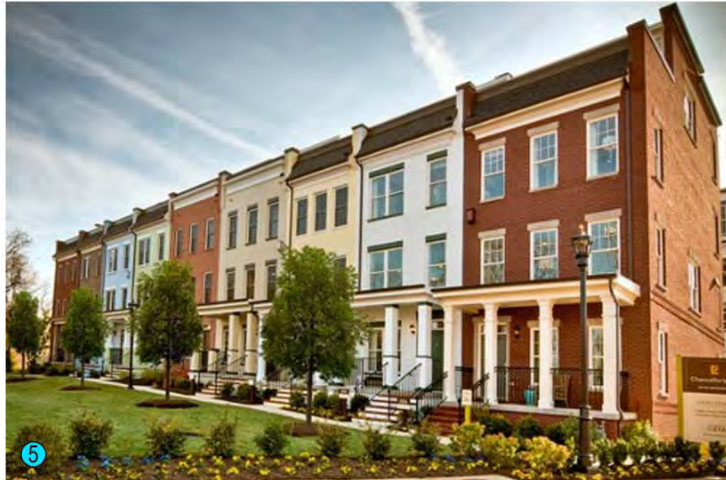
INTERSECTION OF JACKSON STREET N.E. AND REGENT PINE N.E. AT CHANCELLOR'S ROW TOWN HOMES
