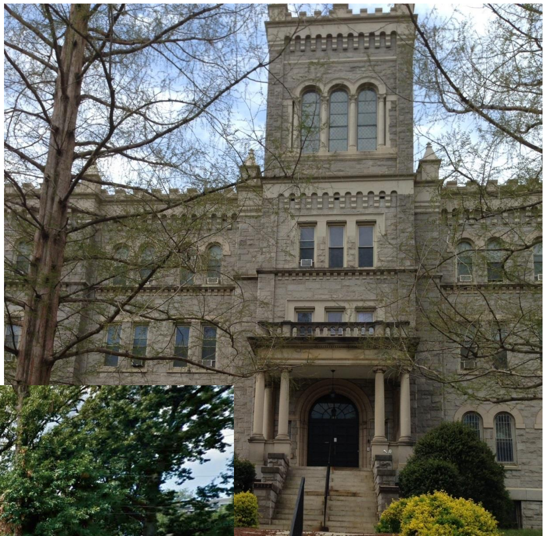
Holy Redeemer College Existing Front
