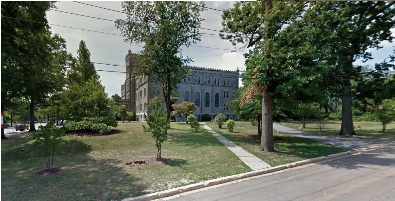
Holy Redeemer College Existing North Façade
