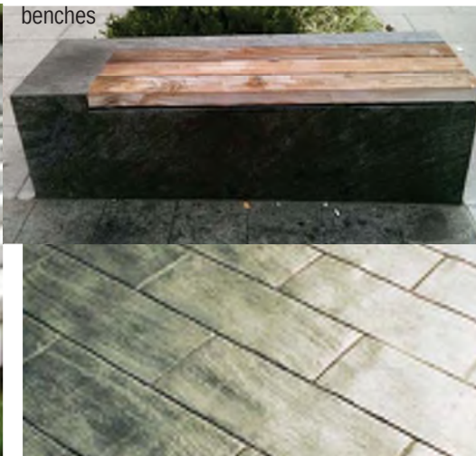
stamped concrete on ADA path
