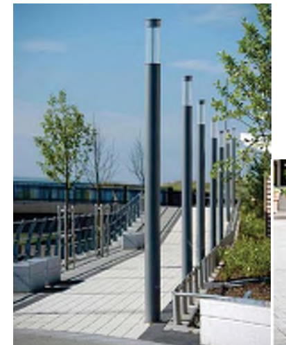
park lighting fixtures
