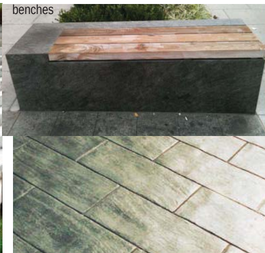
stamped concrete on ADA path
