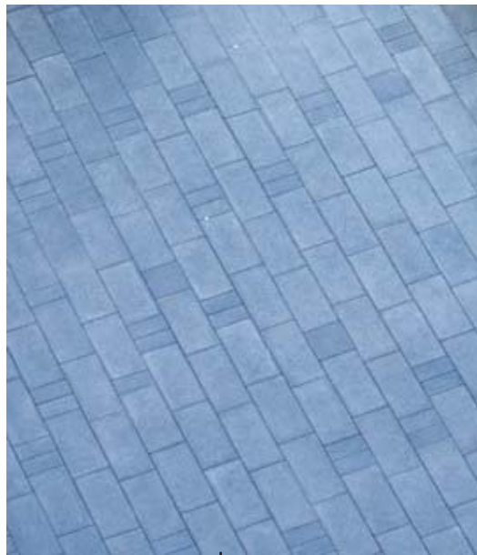
special stone paving
