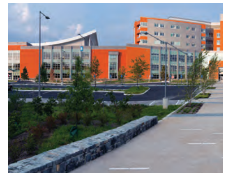
Fort Belvoir Community Hospital, Fort Belvoir, VA
