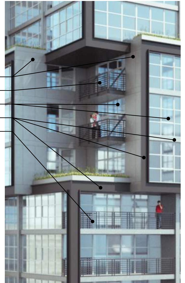
UPPER SOUTH / EAST BUILDING CORNER
