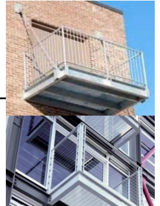
STEEL BALCONY / RAILING
