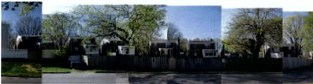
Exhibit 4-155: Looking south along Aspen Street: View of the back of single-family homes in between Luzon Avenue and 13th St.
