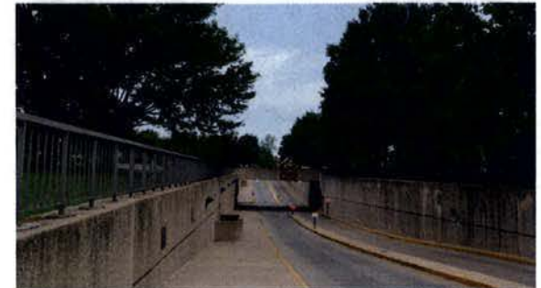
Figure 3-64: Parking access ramp on Georgia Avenue side of the garage. Source: Perkins+Will.
