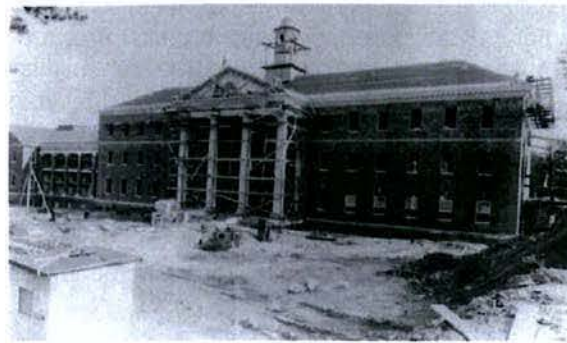
Figure 3-60: View of Building 11 under construction, dated April 8, 1931. Source: National Archives and Record Administration, SC 590550.
