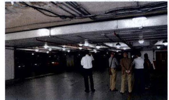
Figure 3-65: Parking garage interior. Source: Perkins+Will.
