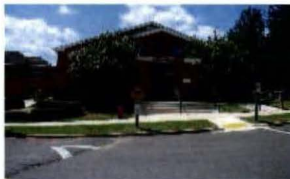
Figure 3-67: View of the entrance to the Child Development on the east end of building 88.
