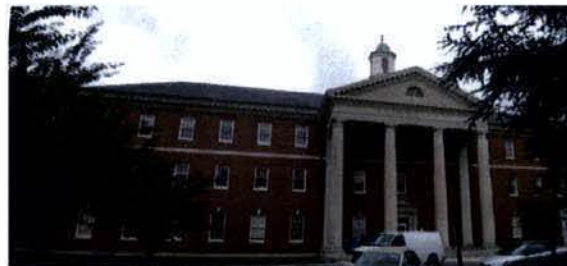
Figure 3-61: View of Building 11 under construction, dated May 2010. Source: Oehrlein & Associates Architects.
