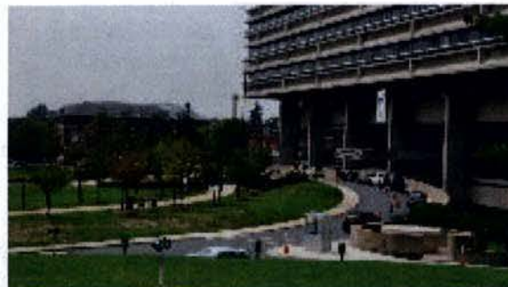
Figure 3-63: Building 2 and the west end building 4 which is the green roof of the parking garage. Source: Perkins+Will.
