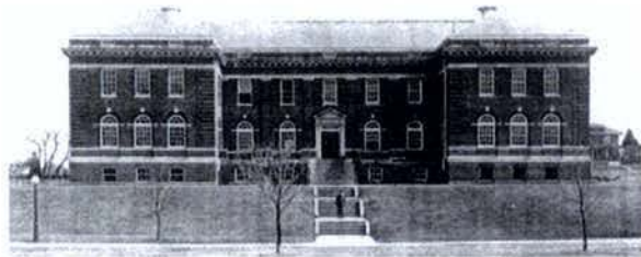
Figure 3-53: View of Building 7, dated circa World War I. Source: Walter Reed Directorate of Public Works Archives, Box #1, Folder #12, 09-4673.
