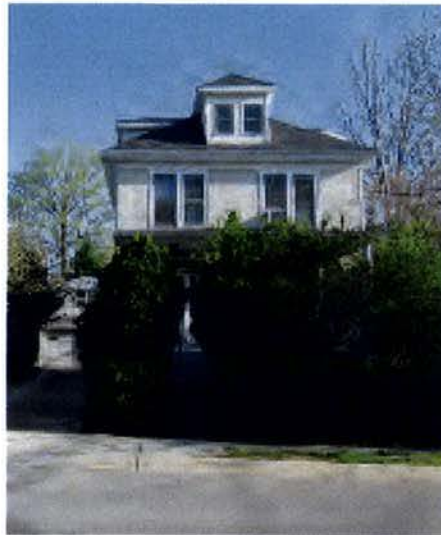
Figure 4-95: View looking north along Fern St. at a three-story residence just east of 13th St. Source: Perkins+Will.
