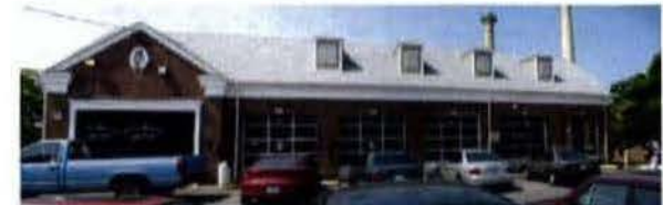
Figure 3-47: View of front elevation of Building 82, dated May 2010. Source: Oehrlein & Associates Architects.
