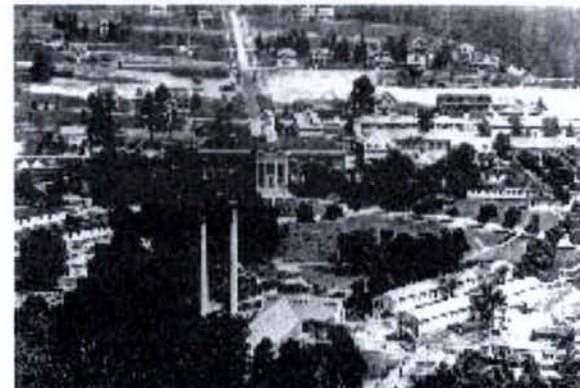
Figure 3-39: 1915-22 Historic Aerial Photo from South View looking north with powerhouse, original bandstand and temporary buildings in the foreground. Source: Walter Reed Directorate of Public Works Archives, Box 1, Folder 1, #09-4467
