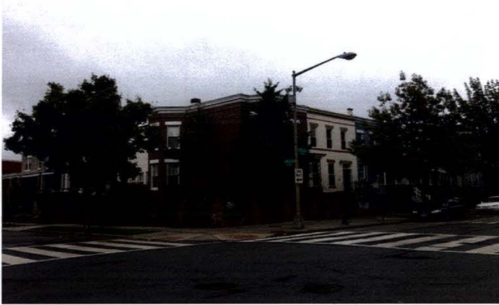
Photo # 2 - View of the intersection at 15th and A Street, NE -- a portion of the "Northwest Quadrant" of Square 1070.
