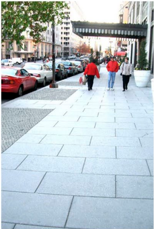
PAVING - 2X3 CONCRETE PAVER
