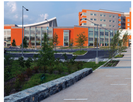
Fort Belvoir Community Hospital, Fort Belvoir, VA
