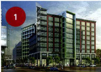
HALFSTREET, 25 M STREET SE - MIXED USE BUILDING
