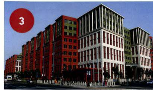
USDOJ HEADQUARTERS, 1200 NEW JERSEY AVE SE
