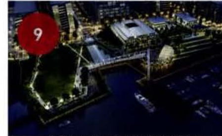
9 THE YARDS PARK, 355 WATER STREET SE - MIXED USE DEVELOPMENT
