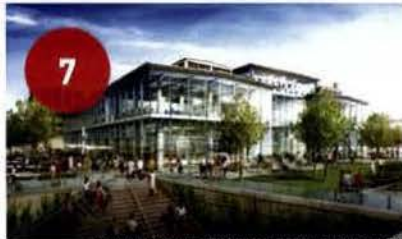
7 THE LUMBER SHED, 301 WATER STREET SE - RETAIL BUILDING
