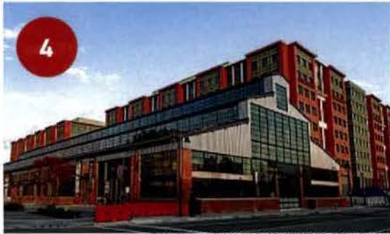
4 THE BOILERMAKER SHOPS, 300 TINGEY STREET SE - RETAIL BUILDING
