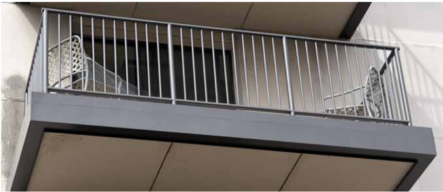
ALUMINUM COMPOSITE MATERIAL (ACM) TRIM AT BALCONIES
