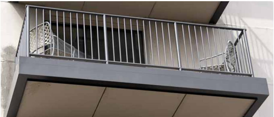
ALUMINUM COMPOSITE MATERIAL (ACM) TRIM AT BALCONIES
