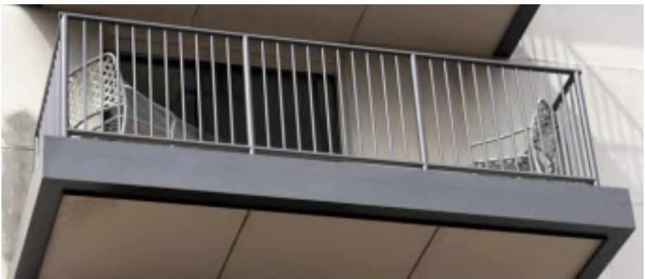
ALUMINUM COMPOSITE MATERIAL (ACM) TRIM AT BALCONIES
