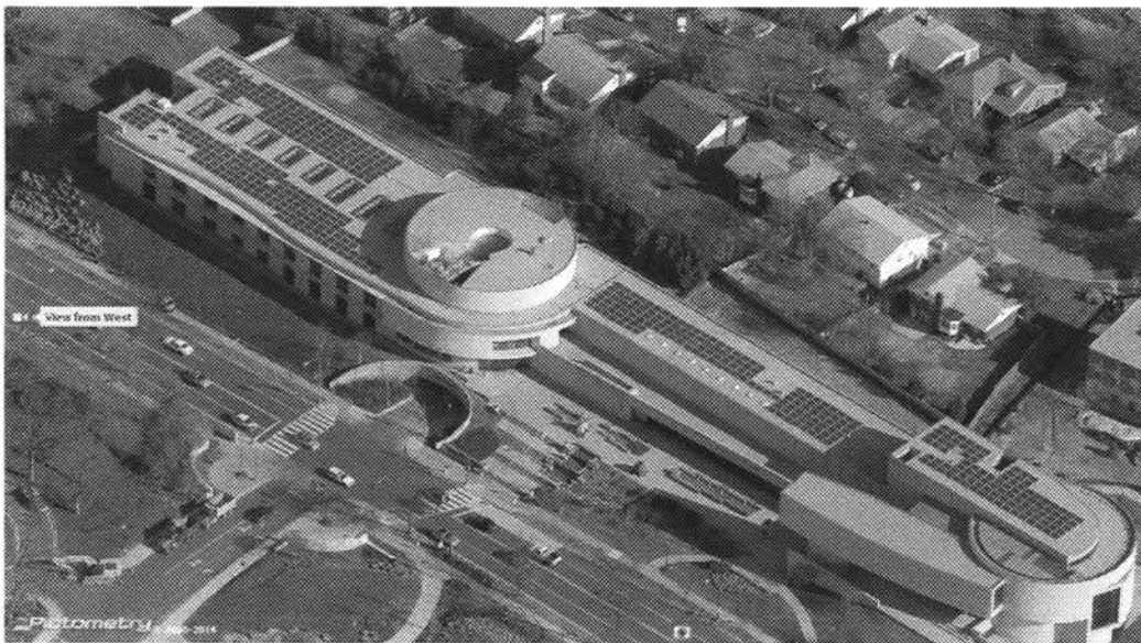
Katzen Arts Center - Solar PV on penthouse, bottom right
