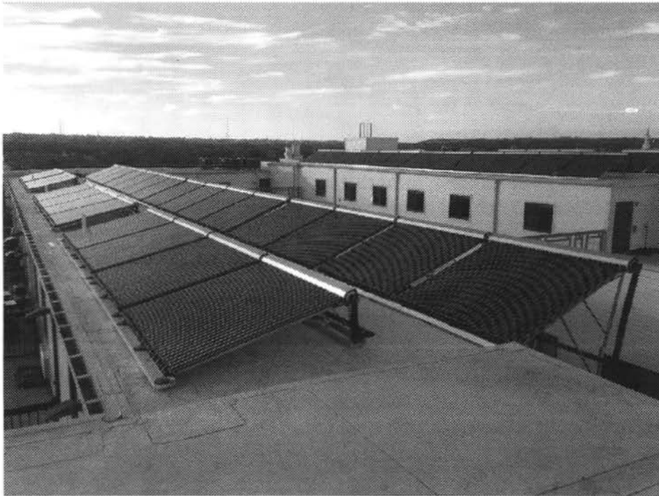
IMAGE 2: Domestic Solar Water Heating System at 3 Tree Flats, a multi-family, affordable housing building in Petworth, DC. System installed by Nextility, a DC company. Note the different slopes and racking systems required for the installation.
