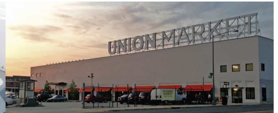
UNION MARKET EXISTING SITE
