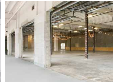
DOCK 5 (exterior to interior)
