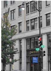
PENDANT STYLE WASHINGTON GLOBE- TO REPLACE EXISTING COBRA FIXTURE (L STREET N.W.) NOTE: SUBSTITUTION REQUIRES DDOT REVIEW AND APPROVAL
